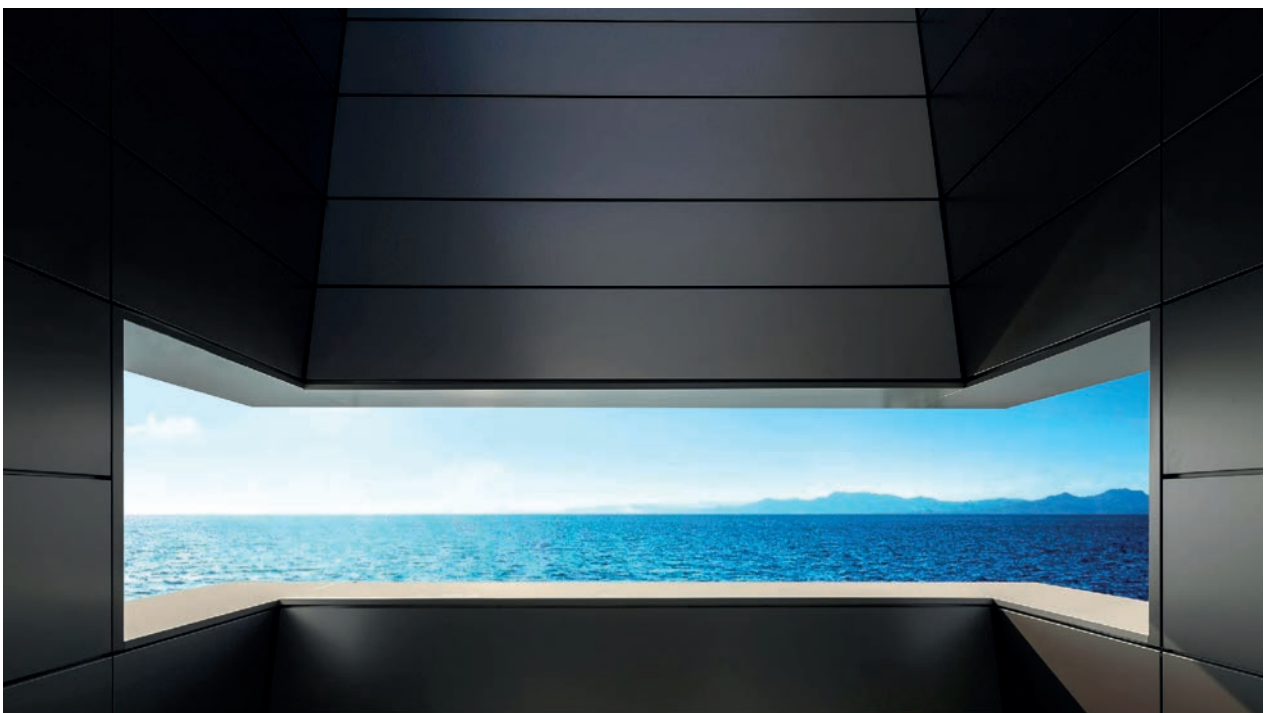
Dock of nautical services | Valencia, Spain
